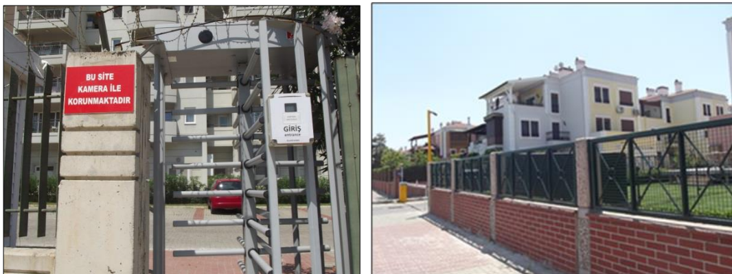
Figure 5, 6: Views from Mavişehir 2st Etape (left figure) and Mavişehir villages (right figure)
