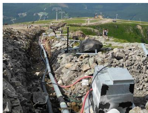
Figure 14. Construction of the new cablecar to Chopok – FUNITEL
