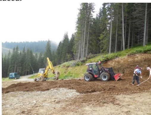
Figure 13. Construction of the new cablecar to Priehyba
